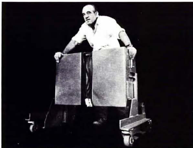
Suggest Safety! Public servant Manfred Moll received $475 for proposing this safe and efficient frame for moving around 500-lb. rechargeable batteries.
