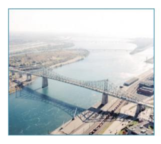
The main span, of a cantilever type, is situated approximately 66 meters above the surface of the St. Lawrence River thus allowing for the passage of vessels to the Port of Montreal. As for the section situated over the St. Lawrence Seaway, it is approximately 49 meters above the surface of the canal.
