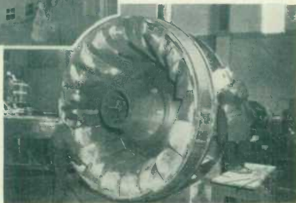
Repairing a Large Turbine Runner by Electric Arc.
