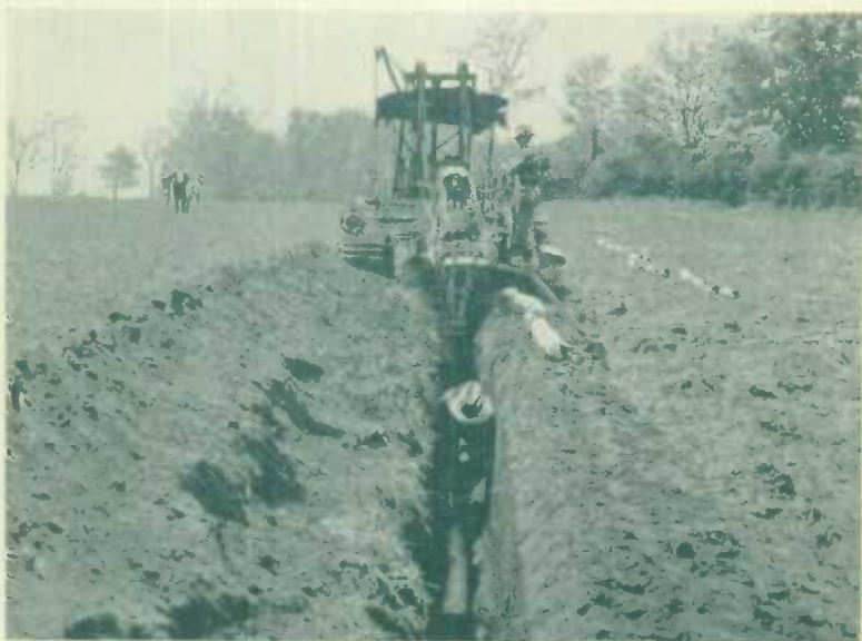
Traction Ditcher at Work. —The under-drainage of farm land is a type of investment which repays the initial cost many times over in increased fertility.
