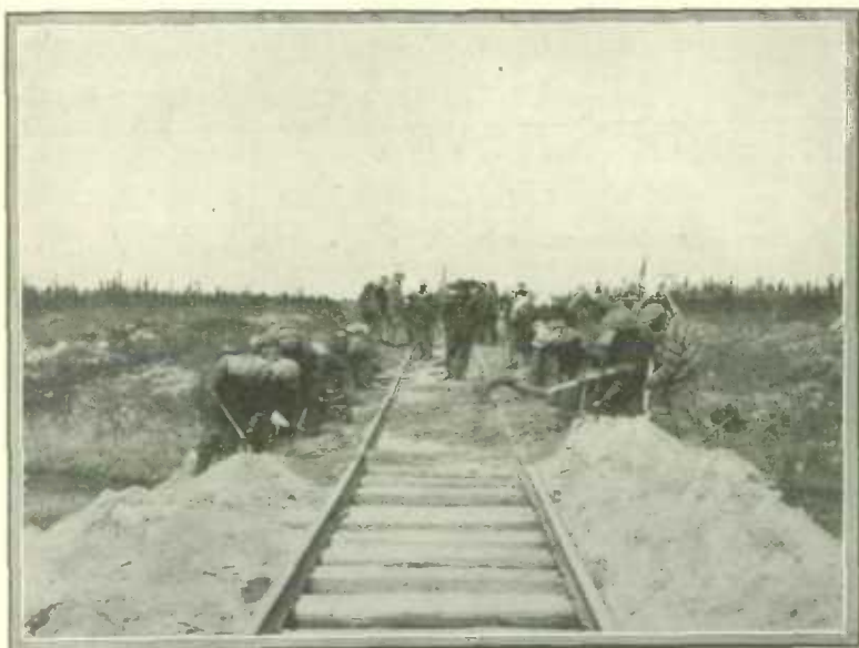
Ballasting a Section of Railway Roadbed.
