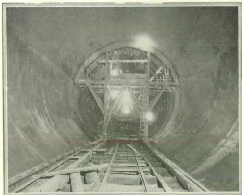
Running Concrete Lining in a Tunnel.—This tunnel, part of the hydro-electric power development of the Lièvre river, P.Q., is 28 ft. inside diameter and over a mile long.
