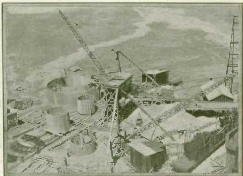
A Mine Shaft Being Put Down Through a Slime-filled Lake. Kirkland Lake District, Ont.
