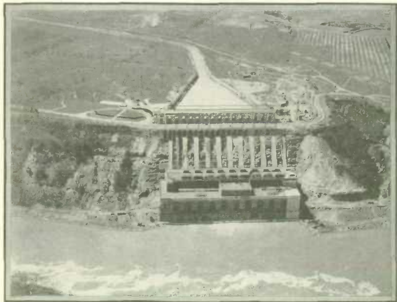
Chippewa Plant, Queenston, Hydro-Electric Power Commission of Ontario.— Installation 560,000 h.p., average head 305 ft. The concrete embedded steel pentstocks shown running down the face of the cliff convey the water from the intake canal to the generators in the power house below. Power is distributed over the Niagara system of the Hydro-Electric Power Commission. This is one of the largest power developments in Canada.
