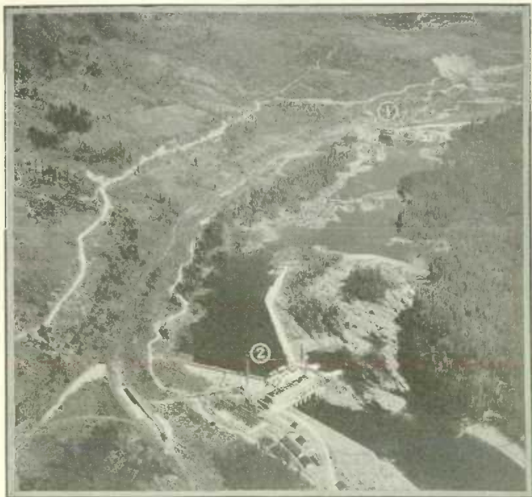
(1) Lower Bonington Falls, 60,000 h.p., and (2) South Slocan, 75,000 h.p. generating stations of the West Kootenay Power and Light Company, Ltd., on Kootenay river. . These stations are inter-connected with two other large plants on the same river to supply the Nelson and Boundary Districts of British Columbia.
