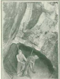
Drilling into the Ore Body in a British Columbia Gold Mine. The lighter vein structure of gold quartz is clearly discernible.
