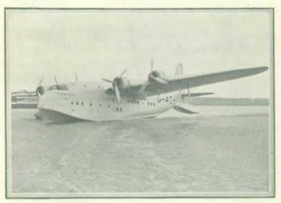
The picture shows the first Empire Flying Boat which has recently gone into service on the Meditorranean route. It has a top speed of about 200 m.p.h. and carries a weight, when fully loaded, of about 18 tons. Extensive experiments are now under way with regard to a transatlantic service by similar boats.
