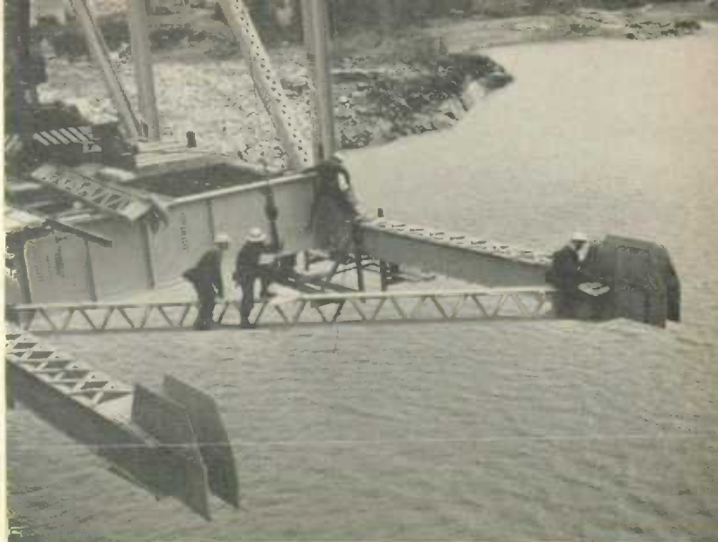
Steelmen riveting girders on a seven-span 1018-foot bridge over the Skeena River, B.C.
