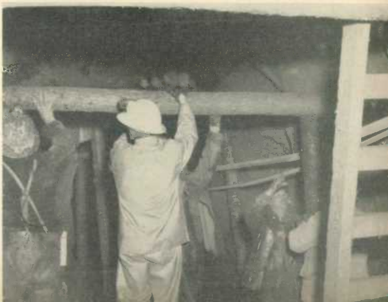
Mine crew placing pit props at the 300-ft. level in the base-metal development at Bathurst, N.B.
