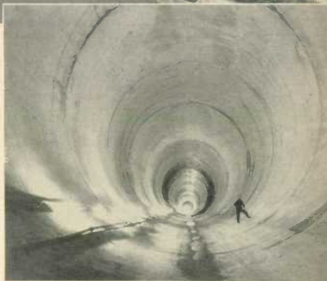
Sir Adam Beck Generating Station No. 2 project on the Niagara River has involved extensive intake works, two 45-foot tunnels 5\frac{1}{2} miles long, two miles of canals, headworks and a power house. Completion is scheduled for 1956.
