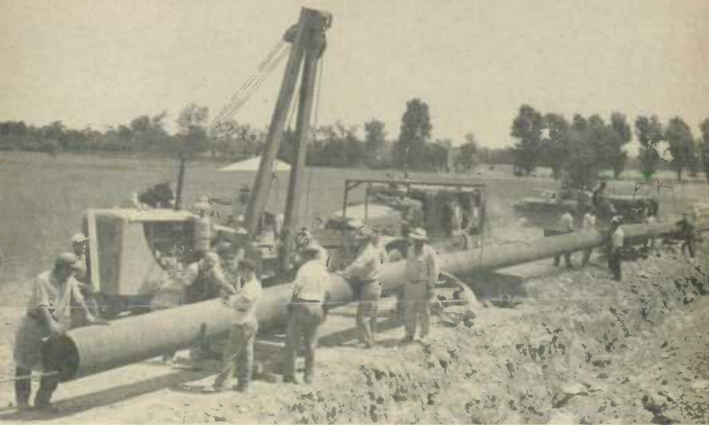
Welding crew working on a natural-gas pipeline running from the International Border at Queenston, Ont., to Toronto. The line, built during the summer of 1954, will carry United States gas to Toronto.
