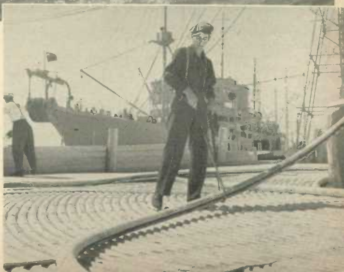
The longest high-voltage submarine cable ever laid carries power from the north shore of the St. Lawrence River to the south shore east of Rimouski, to serve the Gaspé peninsula. Initial power from the Manicouagan River will be replaced by power from the Bersimis plant when completed. The cable was laid on July 29, 1954.
