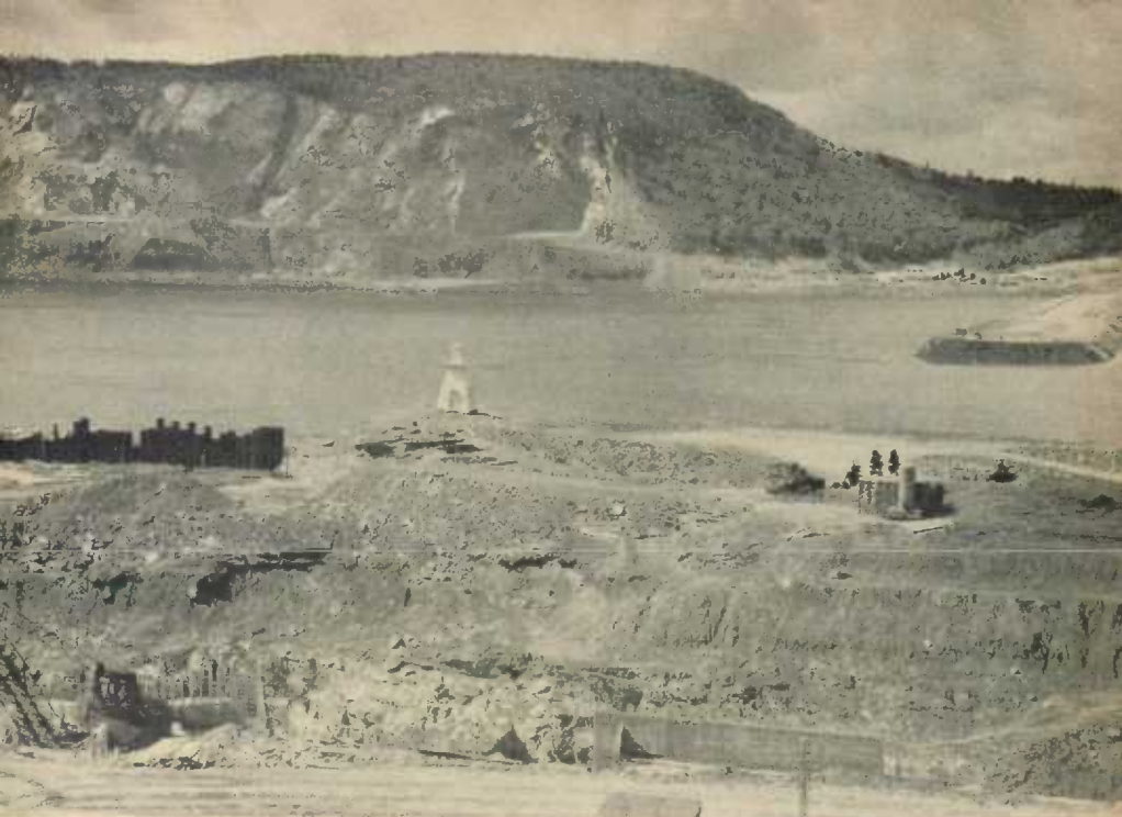
The construction of a causeway across the Strait of Canso will provide land passage from Cape Breton Island to the mainland of Nova Scotia. The causeway, a mile long and 80 feet wide at the top will reach shore just left of the lighthouse. In the foreground is the excavation for the ship channel.
