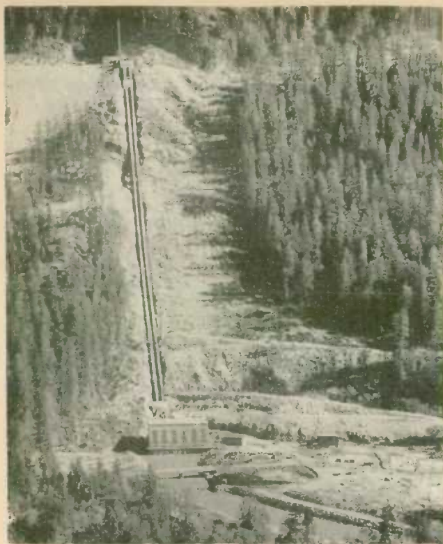
The construction of the power project at Cheakamus, about 65 miles north of Vancouver, was an outstanding engineering achievement—one of the largest remotely controlled hydro-electric plants in the world. It involved the turning of a glacial stream at right angles to flow through a seven-mile tunnel and down 900 vertical feet to the powerhouse. The completion of this project in December 1957 added 180,000 h.p. to British Columbia's power output.
