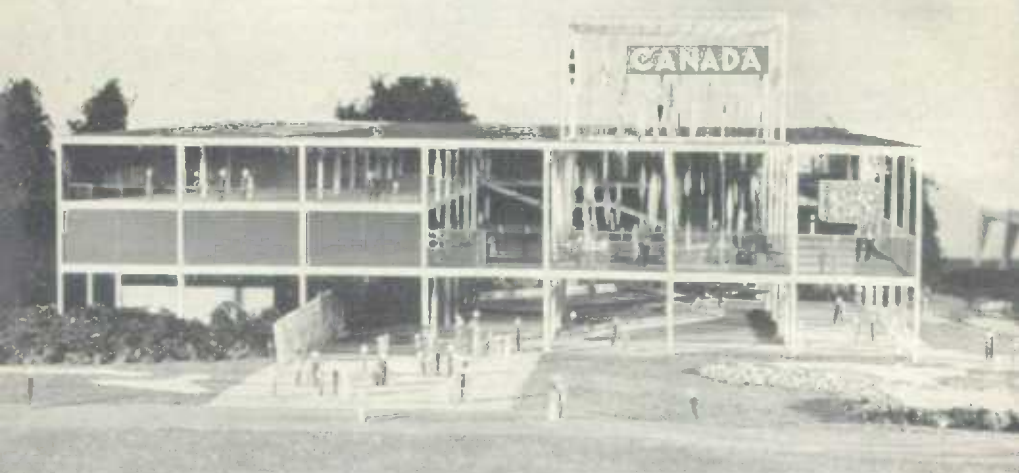
The Canadian Pavilion at the Brussels Universal and International Exhibition, being held from April to October in 1958, was designed to give a sense of spaciousness and relaxation. It is a three-storey building with a white steel frame, constructed of two-tone grey glass and cobalt-blue masonite, and in it the visitor will find many ingenious exhibits portraying the life and work of the Canadian people—their government, their resources, their industrial, social and cultural development.
