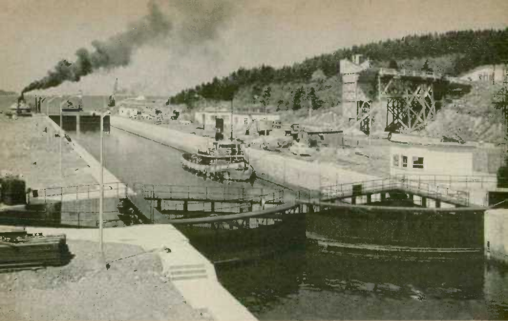
The new Canso Canal between the mainland of Nova Scotia and Cape Breton Island permits vessels northward bound to the Gulf of St. Lawrence or southward bound to the East Coast of Nova Scotia to use Canso Strait and save half a day's sailing time.
