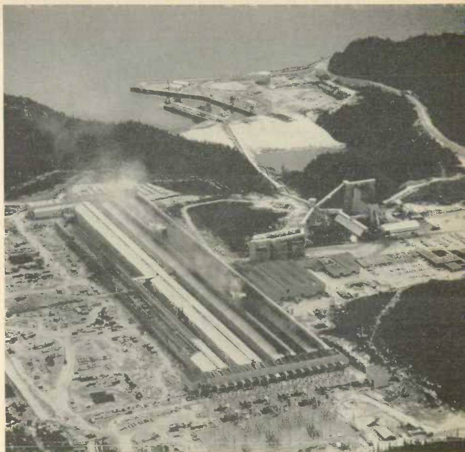
The second stage of construction is nearing completion at the aluminum smelter at Baie Comeau on the north shore of the lower St. Lawrence River. The plant has been in operation since early 1958 but the new addition will increase its annual capacity to 90,000 tons.
