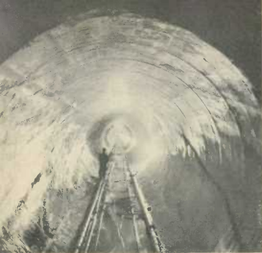
A two-mile hydraulic tunnel will carry water to the Silver Falls plant now under construction on the Kaministiquia River, 30 miles northwest of Fort William. The plant will be in operation in 1959.
