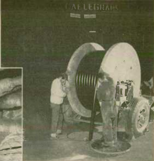
A splicer joining its 5,454 wires—this is the largest cable available to the communications industry today.
