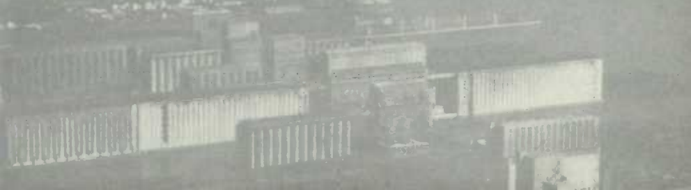
Two control dams have been constructed—the Long Sault Dam and the power plant combine to maintain the head of water required to operate the generators.
