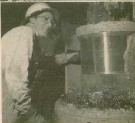
Machining a 3,600-lb. uranium ingot, worth about $50,000.
