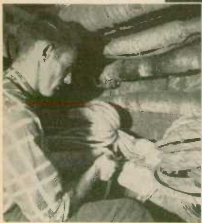
A splicer joining its 5,454 wires—this is the largest cable available to the communications industry today.
