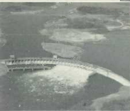
Two control dams have been constructed—the Long Sault Dam and the power plant combine to maintain the head of water required to operate the generators.
