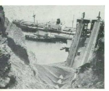
At windswept Bell Island, Newfoundland, iron ore from the world's largest subterranean mine fills seagoing ore carriers at a rate of several tons per minute.
