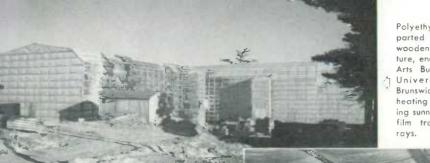
Polyethylene film, supparted by laminated wooden frame structure, enclases the new Arts Building at the University of New Brunswick. No interior heating is needed during sunny days, as the film traps the sun's rays.
