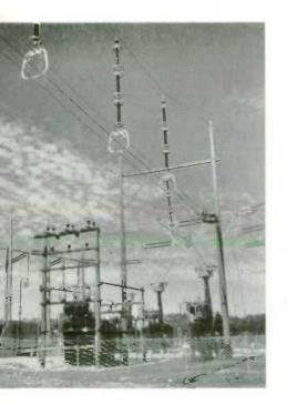
Of importance to the development of far northern rivers are new techniques in high voltage transmission. Ontario Hydro is develaping the first major project of this type in North America. This is the nerve centre of its test line at Caldwater. The three single-phase high-voltage test transformers can be readily identified by the bushing-top instrument houses. They are designed to operate continuously at valtage up to 500,000. The control room is at the lower left.
