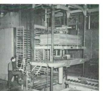
Vaneer lay-sups with an even spread of glue are fed into the hot press. Here a temperature of 285 F, and a pressure of 200 pounds per square inch combine to give plywood its waterproof glue bond.
