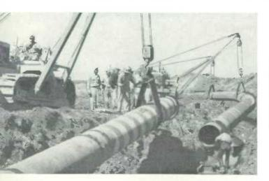
Laying the 51-inch pipeline from Winnipeg to the international border near Emerson, Manitoba. The first gas deliveries through this line to the United States took place is October, 1960.
