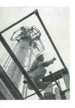
The stripper tower rises above a workman on the naphtha desulphurizer at a Calgary refinery. This unit is the largest addition in a \$1,500,000 expansion program which has increased crude running capacity from 7,500 to 10,000 barrels per stream day.
