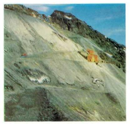
A six-sale coad spaces as McDesse footnate in British Calumbia to the upper levels where asbestos is mined. Mineral is dumped at the upper level, crushed and conveyed dawn to the lower plant where it is loaded into tramline buckets which carry it three miles to the mill at the foot of the mountain. This mine produces obout 40,000 tons of asbestos a year.
