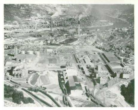
The Trail, British Columbia, operations of the Consolidated Mining and Smelting Company, showing the chemical fertilizer plants in the foreground and the metallurgical operations in the background, which includes the largest zinc plant in the world, producing 530 tons per day of zinc, 400 tons of lead, 1,600 tons of fertilizer plus significant quantities of silver, cadmium, bismuth, gold, ontimony and indium.
