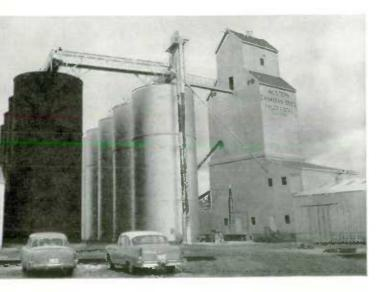
This new oil-seed crushing plant at Lethbridge, Alberta, came into operation in 1960 with an initial capacity of 60 tons of crude oil daily. It also has facilities for seed-cleaning.
