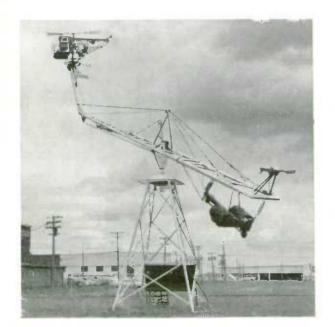
This trainer helicopter rises 75 feet from the graund, can hover, move up or down or sideways, turn on its axis and duplicate the motions of a real helicopter. Used to train pilots in Edmanton, Alberta, it is very much less expensive as a trainer than using a helicopter.
