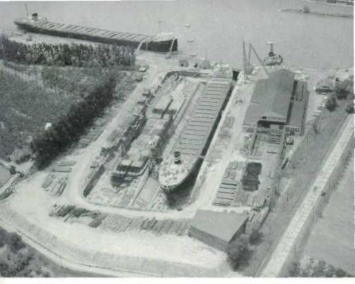
The Port Weller shipyard on the Welland Canal at St. Cathorines, Ontario. Situated in one of North America's oldest ship-building centres, it has a 730-foot building dock, a 750-foot graving dock for repairs and a 100-foot sheerleg crane, the largest ever built in Canada, capable of lifting 125 tons.
