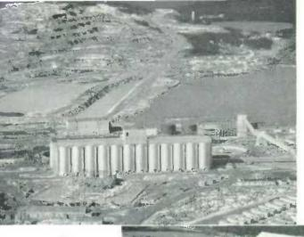
At Port Cartier, near the mouth of the St. Lawrence, a vast half-mile-long hale is being blasted out of solid rock to form one of Canada's deepest harbours which, with a depth of 56 ft., will be able to take 100,000-ton boats to transport iron are brought 193 miles by rail from Lac Jeannine. To build the harbour, 6,500,000 yards of granite must be blasted and shovelled out.
