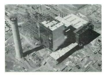
Installation of major equipment at the Nuclear Power Demonstration Station near Rolphton, Ontario, is going ahead. Canada's first nuclear power plant, known as NPD, is scheduled for operation during 1961. It will generate 20,000 kw. and is intended to be used as a demonstration plant to provide a training centre for operators who will be required in the large nuclear pawer plants planned for the near future.
