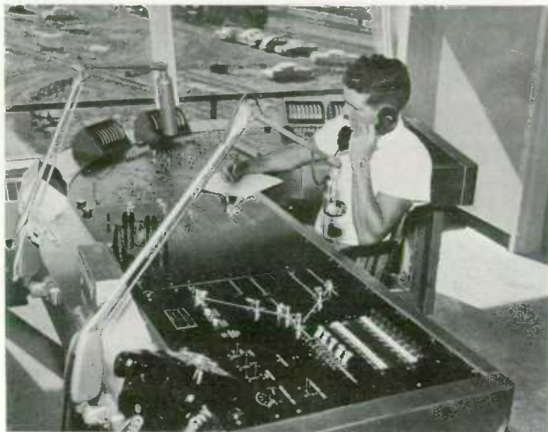
The control console in the retarder tower at the modern $15,000,000 freight marshalling yard at Moncton, N.B., which is equipped with such aids as an electronic brain, integrated data processing, closed circuit television, radar, two-way radio, teletype and tape recorders to speed the sorting of freight cars.
