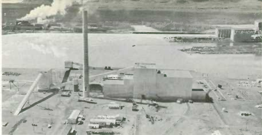
Power was delivered in 1962 by the Thunder Bay Generating Station, the first thermal-electric plant built in the northern part of Ontario. The powerhouse structure approximates the height of an 11-storey building, while the stack rises to 350 feet. The coal-conveying equipment can carry 500 tons an hour from the dock to the stockpile.
