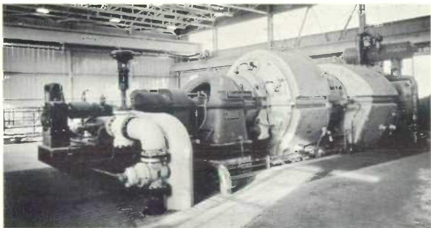
Expansion of capacity of natural gas pipelines is achieved by installation of compressor equipment. This 9,000 hp. unit is one of 13 in operation on the main line carrying gas from the prolific fields of Western Canada to Ontario, Quebec and the United States.
