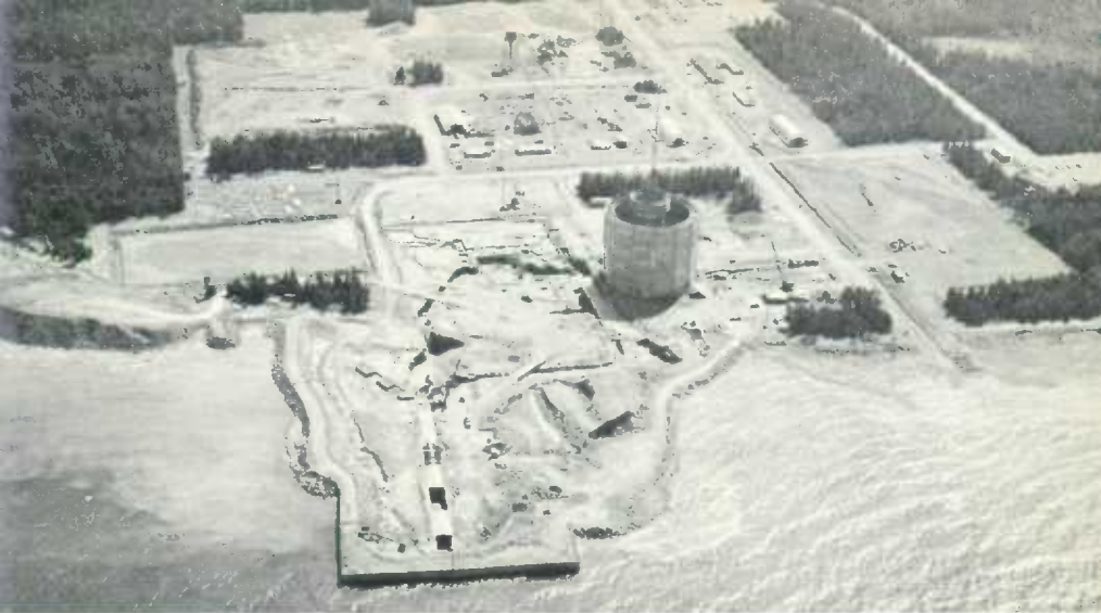
Canada's first full-scale nuclear power station under construction at Douglas Point on the eastern shore of Lake Huron, Ontario. It will have an electrical output of 200,000 kw. when it goes into operation in 1965.
