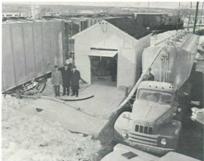
Trans-shipment of dry, granular or powdered commodities from airslide railway car to tanker truck is effected by siphon. At present, flour and sugar are moved by this method, eliminating the costs of bagging and the problems of breakage, wear and leakage.
