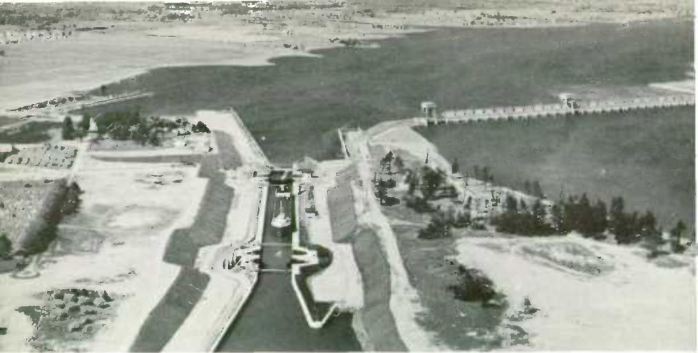
The Iroquois Lock, most westerly of seven new locks built for the St. Lawrence Seaway, enables ships to pass between the power pool or Lake St. Lawrence, at the top, and the Thousand Islands section of the St. Lawrence River, at the bottom, leading upstream to Lake Ontario. On the right is the Iroquois Dam which controls the level of Lake Ontario.
