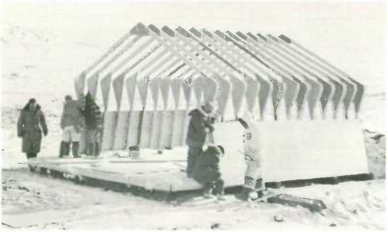
Eskimos at Frobisher Bay on Baffin Island erect a 16' x 16' rigid frame house as part of the Federal Government's ten-year program of providing low-cost Eskimo housing. This model costs about $500 at Montreal.
