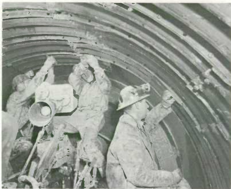
These workmen, working under compressed air, are placing a metal lining in a tunnel bored through clay to house a collector sewer. Later the entire tunnel will be lined with concrete.
