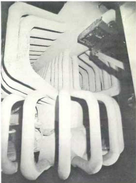
The steam generator in the Nuclear Power Demonstration Station at Rolphton, Ontario.
