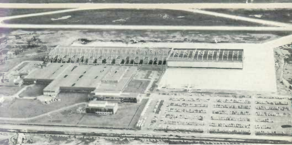
The $20,000,000 engineering, maintenance and overhaul base at Montreal International Airport, the first and largest of its kind designed solely to handle turbine aircraft. The overhaul hangar boasts the largest single cantilever roof in the world; to its right is a double cantilever maintenance hangar.
