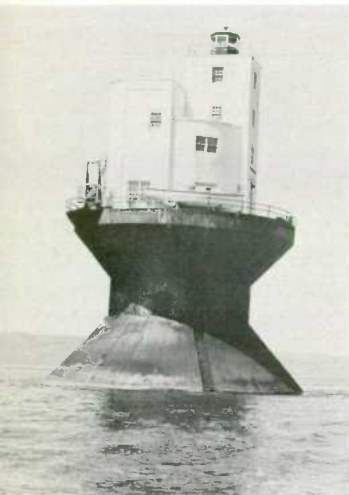
To construct this unique lighthouse at the mouth of the Saguenay River, the caisson was built on land, floated into position, sunk and filled with rocks and concrete. The superstructure was then built.
