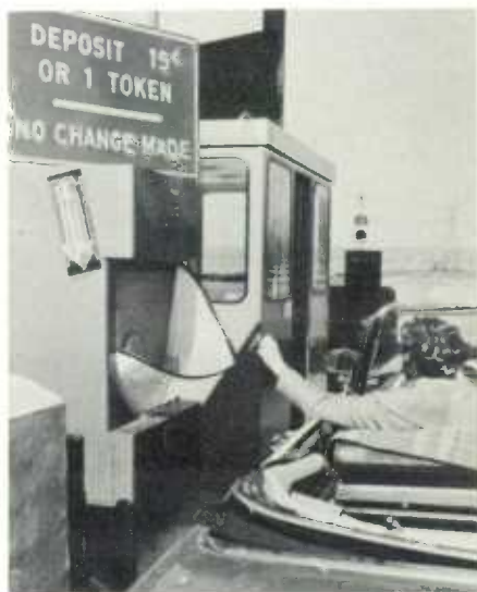
Even collecting tolls is becoming automatic. When a token is tossed into this toll machine, the traffic light ahead changes from red to green and the driver proceeds.
