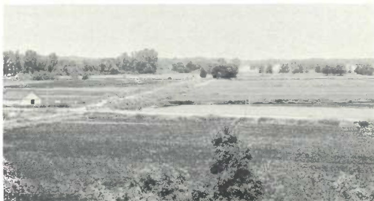
This valuable market garden is growing on reclaimed marshland. Ditches beside the raised roadway provide controlled drainage by which the water table is regulated to prevent flooding or drought.
