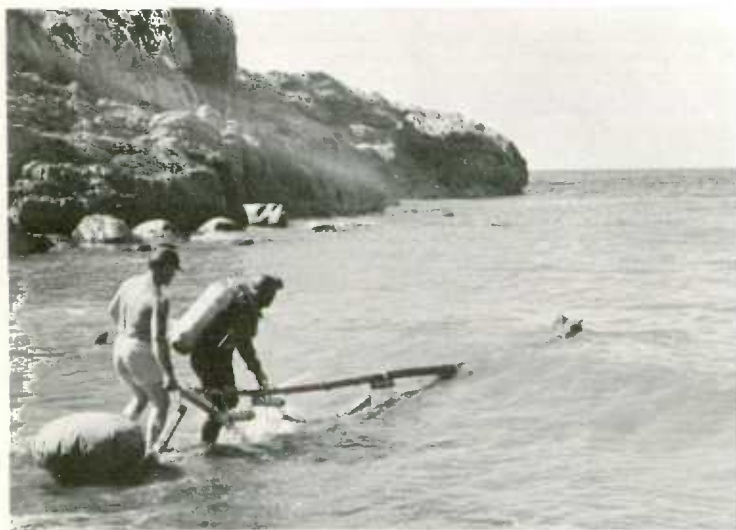
Skindivers lay underwater charges to blast a trench in the sea bed for the transatlantic telephone cable linking Canada and Scotland.
