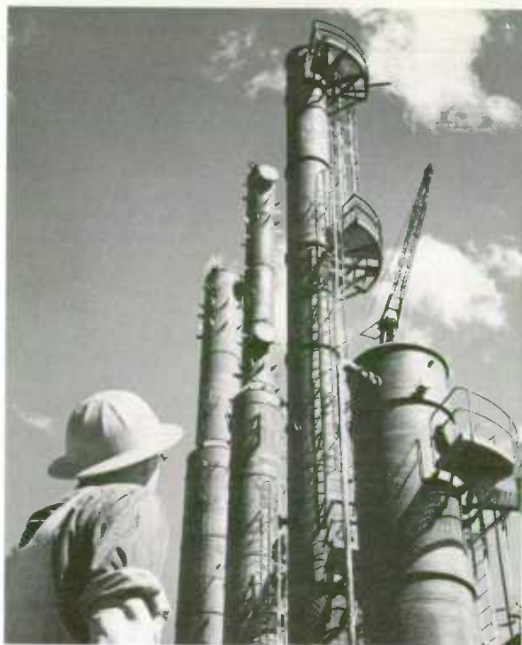
Part of the $5,000,000 gas conservation plant under construction at Judy Creek, 130 miles north-west of Edmonton. Owned by 11 companies, this plant will separate 40,000,000 cubic feet of gas a day, with the natural gas going to Edmonton via pipeline, and the liquified gases going to a gas conservation plant at Devon, where it will be processed into propane and raw materials for industrial plants.
