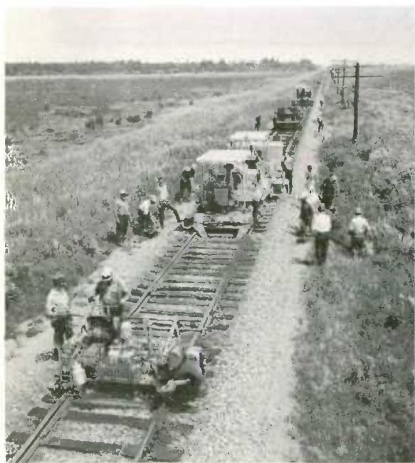
Assembled in sequence of operation are six machines used for replacing ties: in the foreground, the spike-puller; next the dual tie saw; the tie bed scarifier; the tamper jack; the electro-gang-tamper; and the spike-driver. Mechanized tie renewal has cut the labour cost per tie almost in half.
