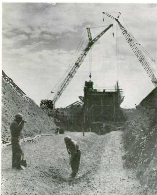
Construction of a sewage settling tank, one of the concomitants of suburban building.
