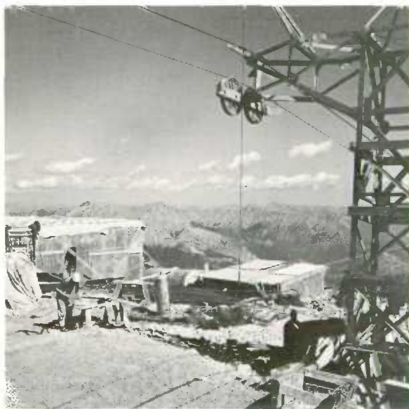
Construction for the microwave system between Grande Prairie, Alberta, and Alaska by the telecommunications departments of the Canadian National and Canadian Pacific Railways involves the installation of repeater stations on mountain peaks, such as this one in the Rockies at an altitude of 9,000 feet.
