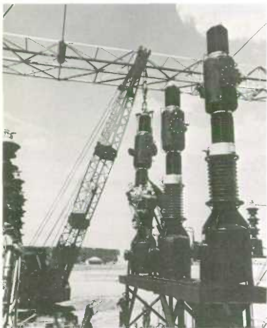
A dramatic photograph of technicians installing circuit breakers.
