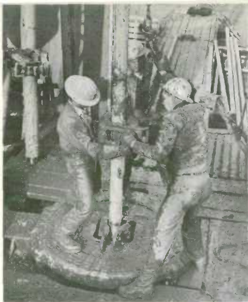
Oil exploration continues unabatedly. Here rough-necks are at work drilling near Wetaskiwin, Alberta.
