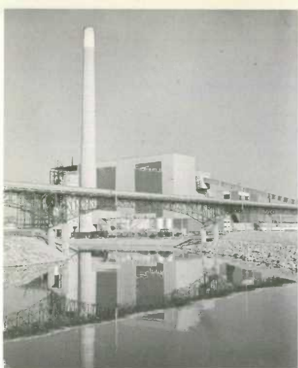
Lakeview Generating Station, where the largest generator of its kind ever installed by a Canadian utility—300,000 kw.—went into production in 1961. By the mid-sixties, when all six units are in service, the $217,000,000 thermal-electric station will have a capacity of 1,800,000 kw.
