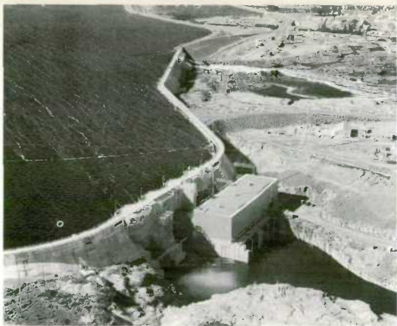
Ontario Hydro's Little Long Generating Station went into production in October, 1963. Located 42 miles north of Kapuskasing, the $48,000,000 station is the first of three plants being built on a 15-mile stretch of the Mattagami River; it has a two-unit capacity of 121,600 kw.
