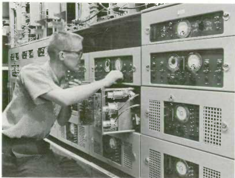
New microwave equipment installed at Fort William in 1962 increased the capacity of the Trans-Canada microwave system by 600 voice-circuits.
