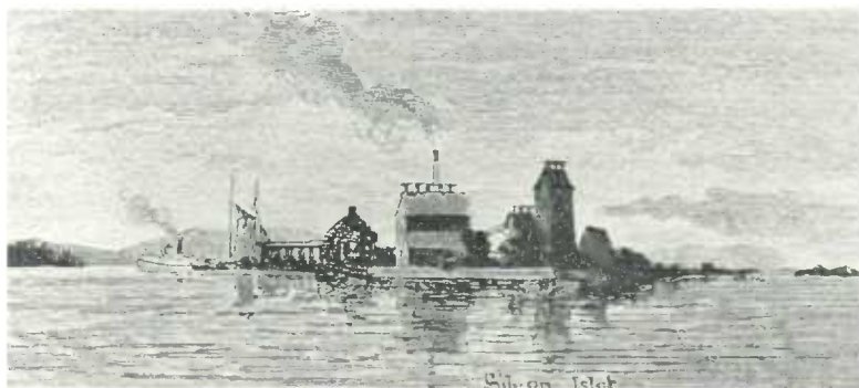
Silver Islet, a tiny island in Lake Superior, originally between 80 and 90 feet in diameter and only about 8 feet above lake level, was Canada's first major source of silver. Between 1868 and 1884, some 3,000,000 troy ounces were recovered in the plant shown in the drawing.
