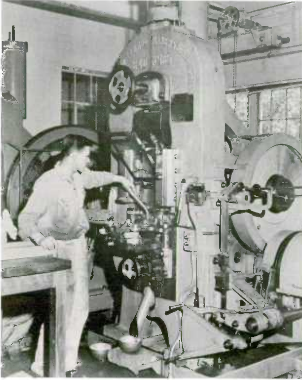
At the Royal Canadian Mint, coin blanks are put into this machine and stamped on both sides. The finished coin drops out the bottom into the little bowl.
