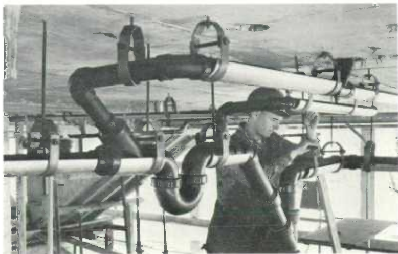
The steady stream of new building produces a demand for heating, electrical and plumbing components. Here a workman installs goosenecks, elbows and traps made from polyethylene.
