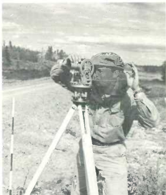
A surveyor works with a transit as he lays out new roadways during the Mackenzie Highway construction in the Northwest Territories.
