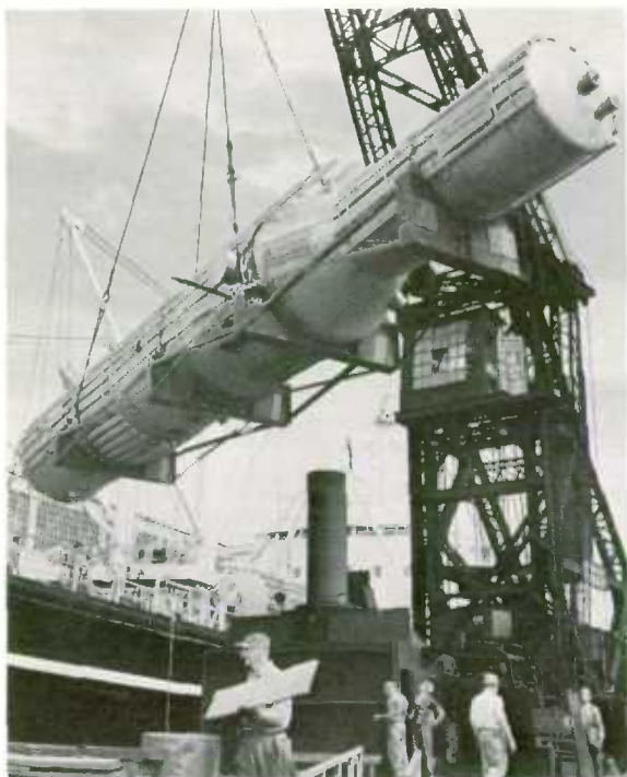
Loading this 58-foot long, 85,000 - pound unit posed a major problem for Montreal's stevedores. It is a process tower with 30 miles of intricately wound copper tubing inside it, part of cryogenic processing equipment to be installed in Algeria to liquefy natural gas from Sahara Desert wells.
