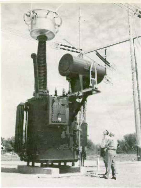
One of the three single-phase high-voltage test transformers now being used in experiments at Ontario Hydro's extra-high voltage test line at Coldwater. Entry into the field of extra-high-voltage transmission was undertaken to develop power sites on the Abitibi and Mattagami Rivers to meet the increasing demands in southern Ontario. The new line will carry 500,000 volts.
