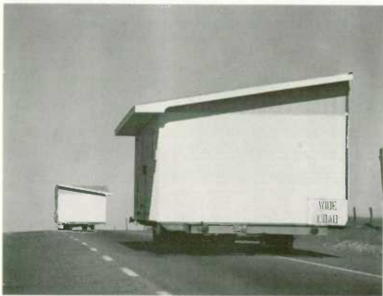
Two halves of a housing unit, part of a large convoy, begin their long journey from Calgary, Alberta, where complete portable housing facilities are made to order.
