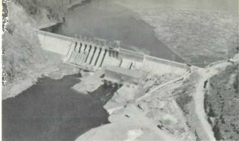
Ontario Hydro's Red Rock Falls' generating station has a capacity of 40,000 kilowatts from two units. This $19.1 million project is located on the Mississagi River.
