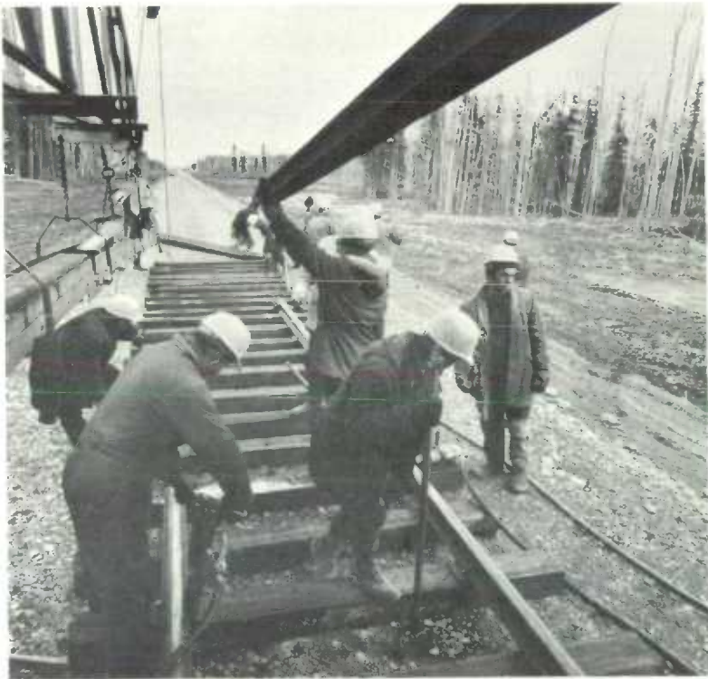
A track-laying crew works on the 430-mile Great Slave Lake railway which runs from Roma, Alberta, to Hay River, Northwest Territories. The line was completed in the fall of 1964.
