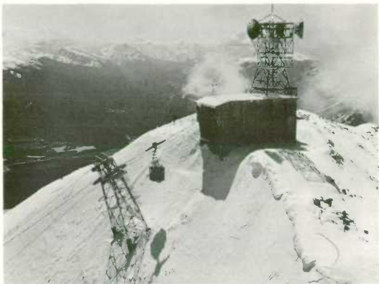
This microwave antenna near Jasper, Alberta, is 9,000 feet above sea level—the highest site of the CN-CP telecommunications Montreal-Vancouver microwave network.
