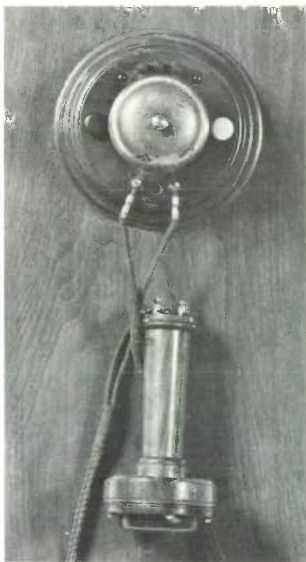
(Above) The new electronic push-button telephone is now in use in a number of Canadian cities. (Right) A telephone used by subscribers to Canada's first telephone exchange which opened at Hamilton, Ontario, in July 1878. The bell was used for signalling and the wooden gadget below for talking and listening.
