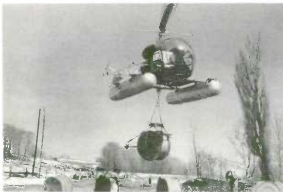
Helicopters prove their worth in hydro line construction. Where the terrain is particularly formidable, the whirly birds fly in pre-assembled sections of aluminum towers and perform other heavy lifting chores. They are also used for line maintenance.
