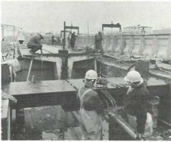
Casting reinforced concrete girders, Saint John, New Brunswick. At the end of 1964, the mileage of highways and rural roads in Canada (exclusive of those in centres of more than 1,000 population) was 438,866.
