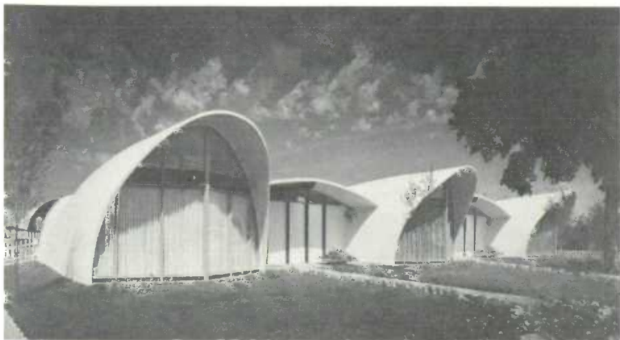
A unique application of plastic in the construction field is this housing unit which was originally designed for the Canadian climate but has since achieved popularity in warmer countries as motel units and homes. The buildings are made of fibreglass and polyurethane foam.
