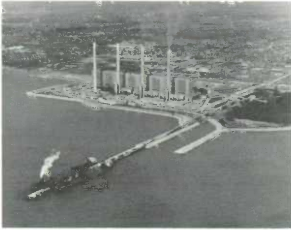
Ontario Hydro's thermal-electric Lakeview Generating Station, under construction on the western outskirts of Toronto, has four 300,000 kw. generators installed at the $268,000,000 plant. By 1968 when eight units are completed, this station will have a capacity of 2,400,000 kw.
