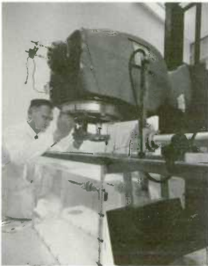
The gamma ray beam in the head of this cancer therapy machine is tested before final assembly. The therapy units service more than 200,000 cancer patients annually in many countries throughout the world.
