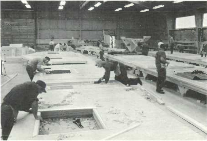
Prefabricating of housing units, as in this plant at Buctouche, New Brunswick, provides for faster on-site construction.
