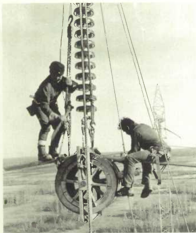
It's a long way down for men stringing conductor for the Nelson River transmission line in Manitoba.
