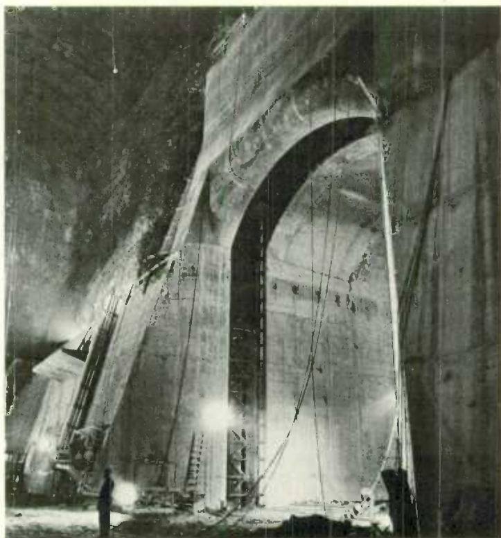
One of the east tailrace inlet portals of the Chardull Falls project, where water from the surge chamber enters the 5,500-foot-long tunnel. The doors measure 60 ft. by 45 ft. wide.
