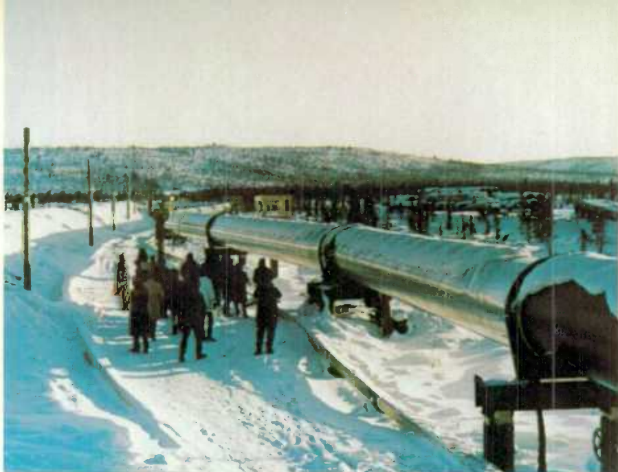
At Inuvik in the Northwest Territories the laying of oil pipeline is tested. The melting of the permafrost must be guarded against.
