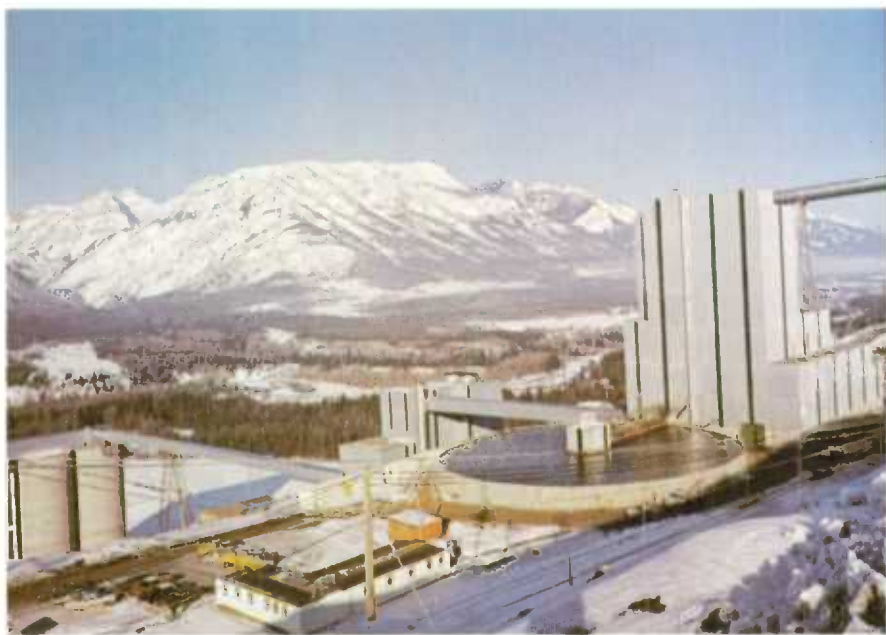
Kaiser's plant in the Elk Valley, B.C. Here coal is washed and dried, then stored for shipment.
