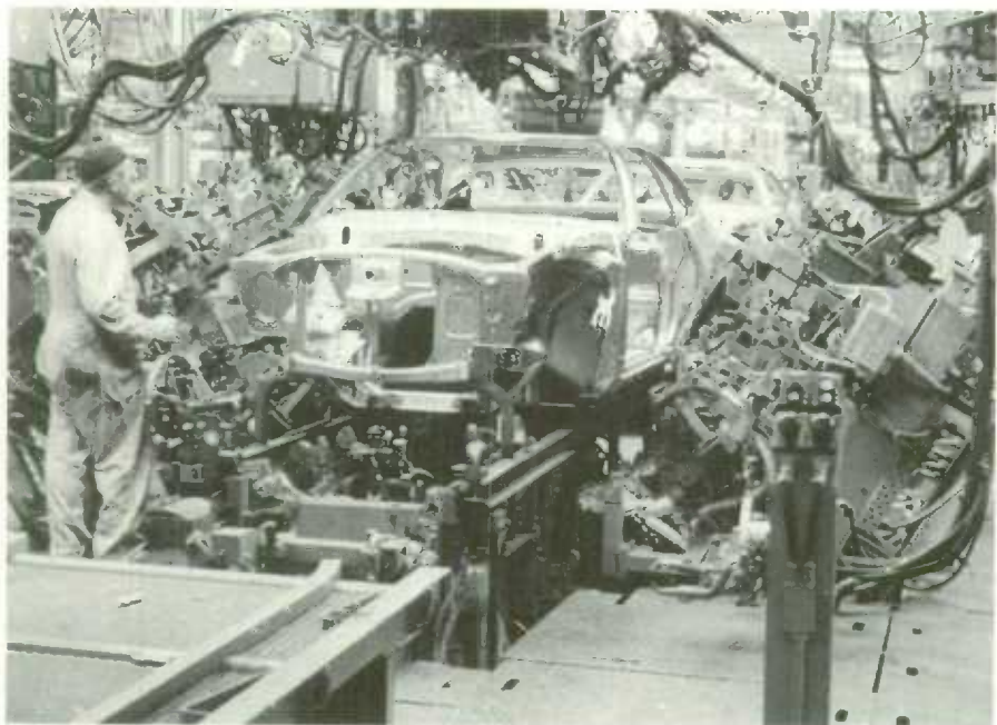
At the push of a button, the automatic pivoting pillar buck—or "Monster" as it is called—instantly applies 135 welds to sub-assemblies and forms a new automobile body.
