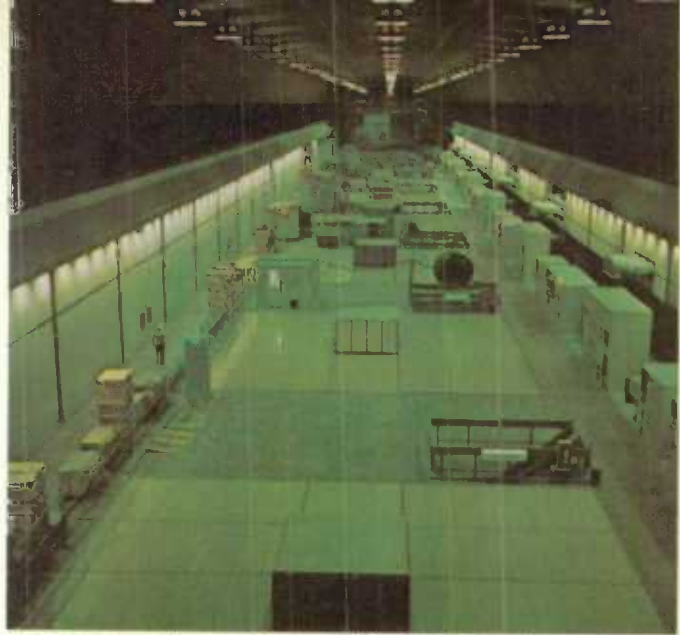
The underground powerhouse (1,000 feet below the surface) at Churchill Falls, Labrador. Upon completion of this hydro project, the capacity of the plant will reach 5,223,000 kw.
