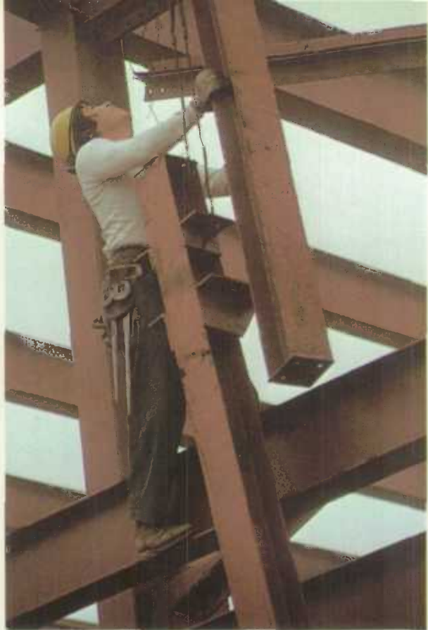
A worker guides a steel beam into place at the construction site of a new department store.
