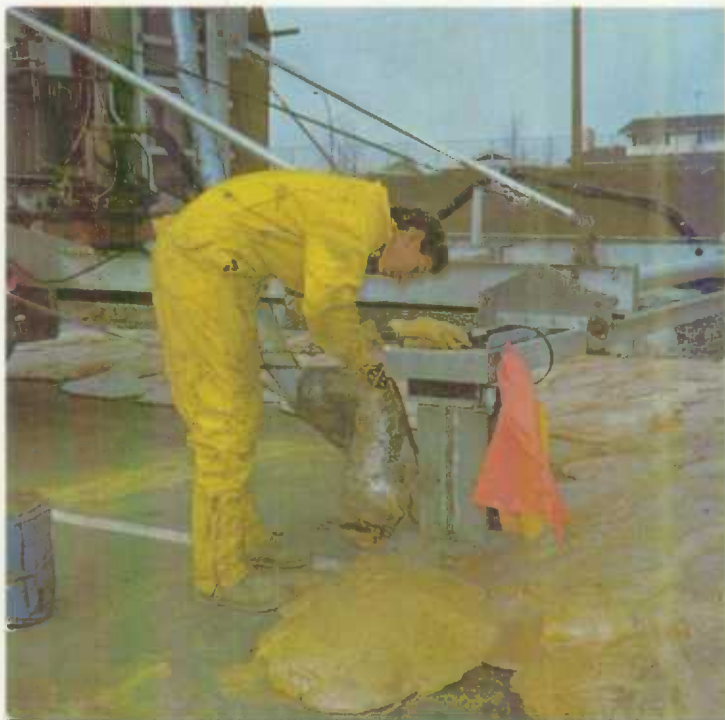
An experiment in Calgary, Alta., aims to determine the value of sulphur as a sub-base for street pavement.
