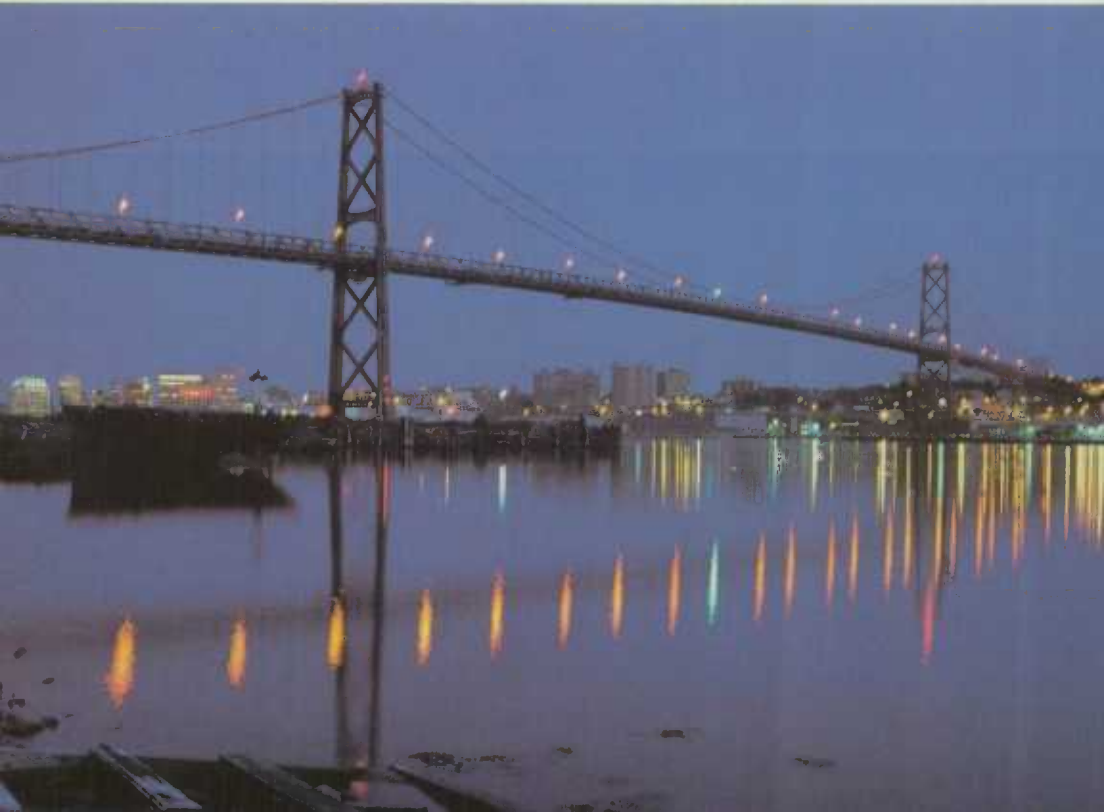
The Angus MacDonald bridge at Halifax, NS.
