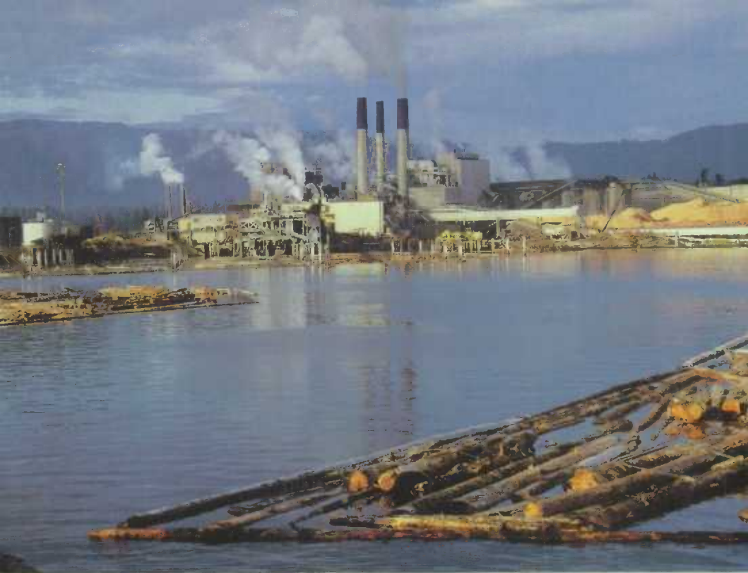
Pulp and paper plant at Port Alberni, BC.
