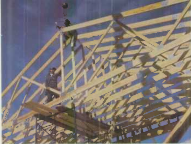
Construction near Vinson, Que.
