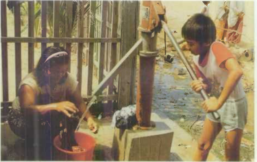
Women and children in developing countries often spend many hours each day collecting enough water for drinking, cooking and washing. IDRC has financed the development of a reliable handpump, such as this pump in Malaysia, that can be easily repaired locally and can be cheaply manufactured in developing countries.
