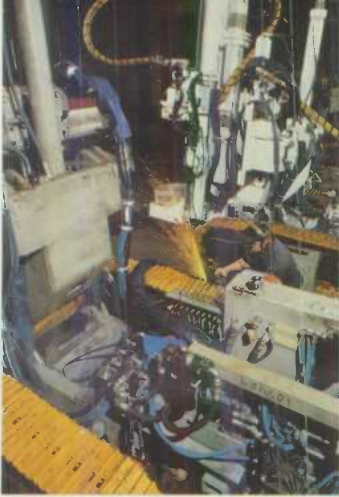
Underground drilling at Continuous Mining Systems in Sudbury, Ont. The new underground drill has gained acceptance in foreign markets, particularly in South America, Australia and China.
