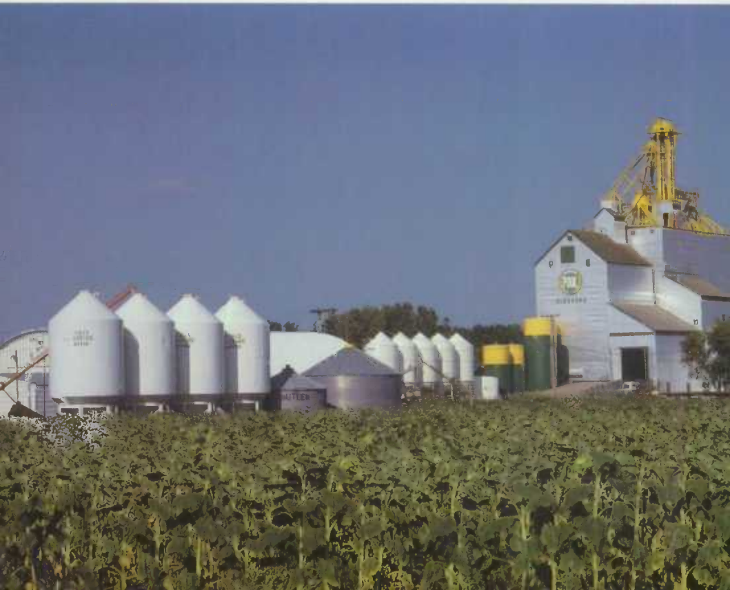
Pool elevator near Glenboro, Man.
