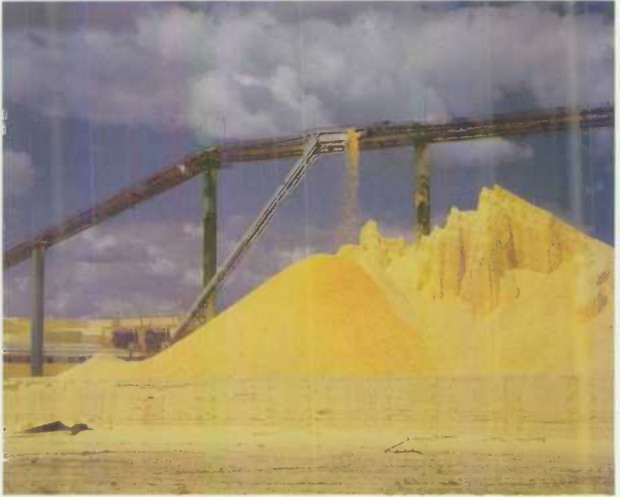
A sulphur recovery plant, north of Calgary, Alta.
