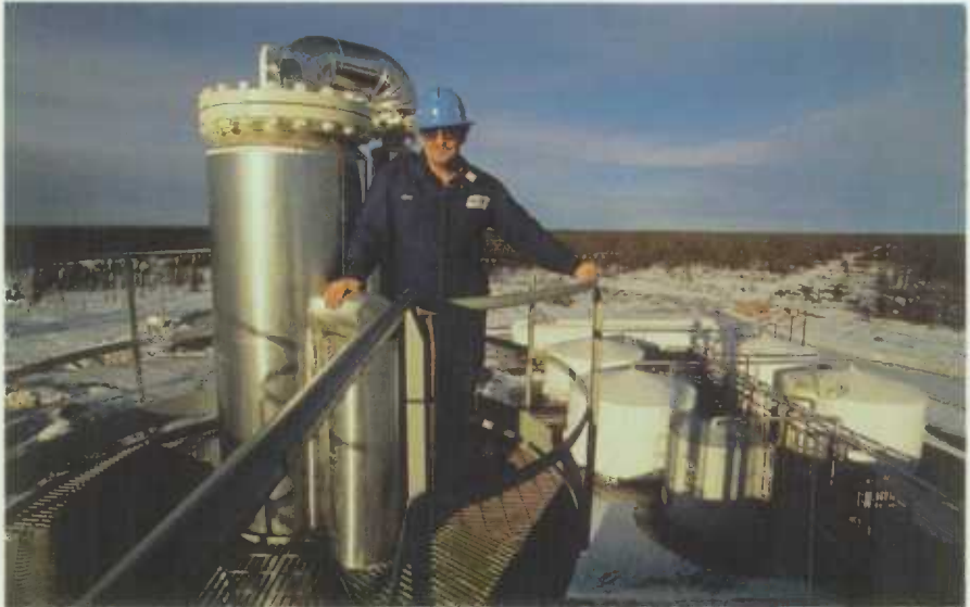
A new seismic oil and gas plant facility at Rainbow, Alta.
