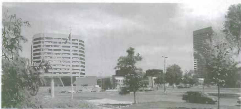
Statistics Canada, Tunney's Pasture, Ottawa From left to right: Jean Talon Building, Main Building, R.H. Coats Building
