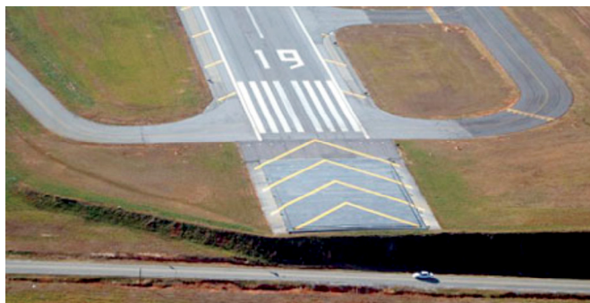
Figure 9.1—Photograph of an EMAS Installation
