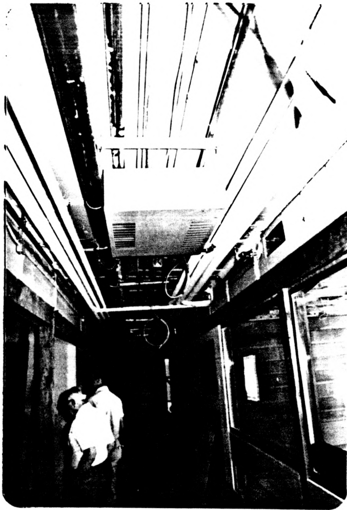
46. FORCE-FLO HEATER IN CORRIDOR CEILING
