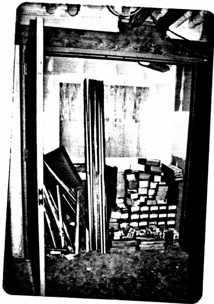
40. TELEPHONE "CLOSET" 130A
