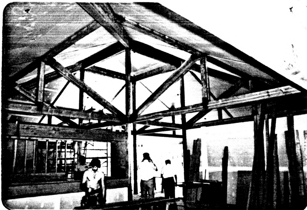
24. ROOF TRUSSES
