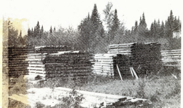
Rough Lumber undergoing Seasoning at Lake site one-half mile from Sawmill
