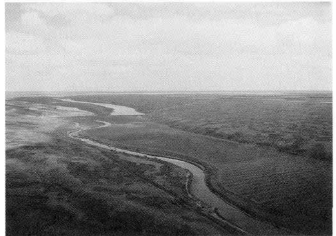
The Midale Dam and Dead Lake looking upstream to the northwest. The sliver of land between Dead Lake Channel and the main Souris River is designated as wildlife mitigation land (photo credit: The SBDA).
