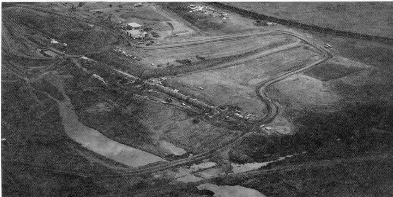
Alameda Dam construction site with the low-level outlet structure in the centre, April 1991 (photo credit: RJ Riewe)
