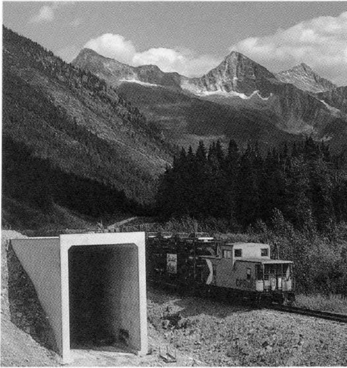
Concerns expressed during the panel review of CP Rail's Rogers Pass project, Glacier National Park, resulted in the relocation of the tunnel ventilation shaft
