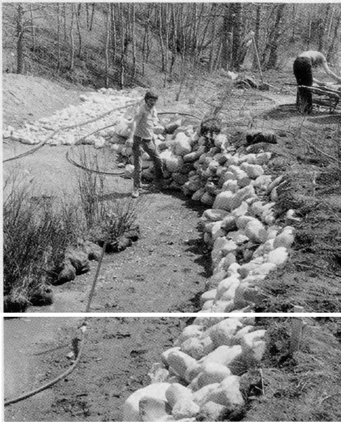
Creek realignment and fish habitat enhancement during the twinning of the Trans-Canada Highway through Banff National Park
