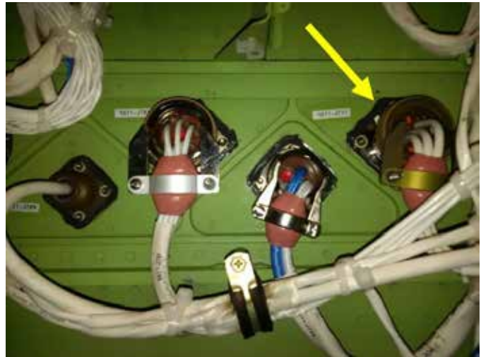
Figure 1. The 9811-J711 electrical connector, indicated by the arrow (Source: Bombardier Aerospace, with TSB annotations)
