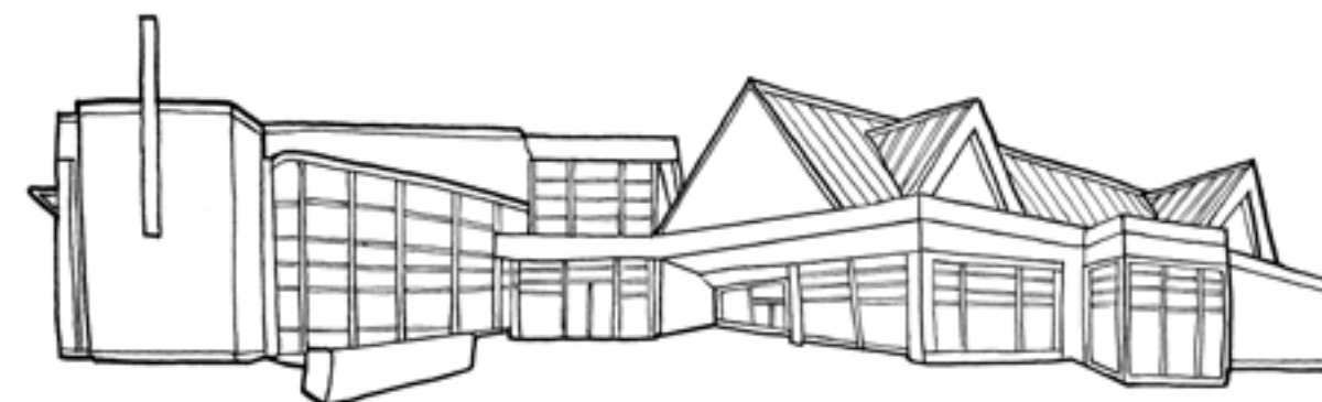
BRAMPTON PUBLIC LIBRARY - CYRIL CLARK BRANCH
