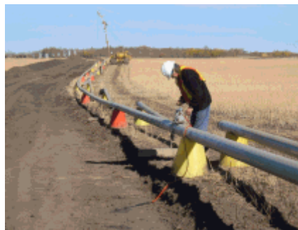
Image 6: NDT Pipeline inspection, using industrial radiography equipment
