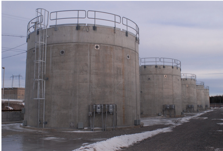
Figure 5.5: Point Lepreau retube waste canisters
