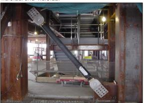
Figure 17: Illustration of supplementary energy dissipation deviceviscous damper
