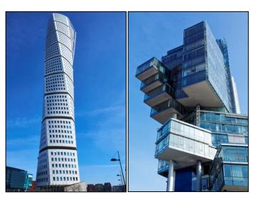
Figure 14: Buildings with gravity-induced lateral demand
