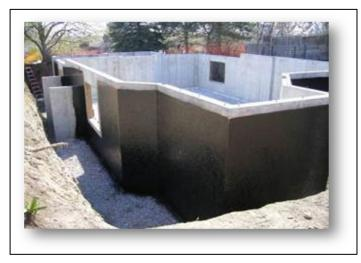
Figure 5: Foundation dampproofing
