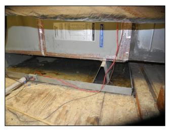
Figure 6: Contaminated drain pan condensate
