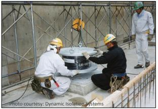
Figure 16: Seismic isolation using lead rubber bearing
