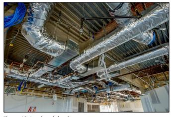
Figure 10: Insulated ducting
