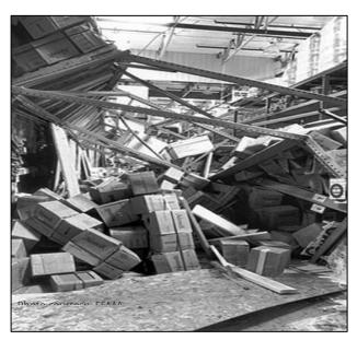
Figure 15: Failure of steel pallet storage racks in Northridge earthquake
