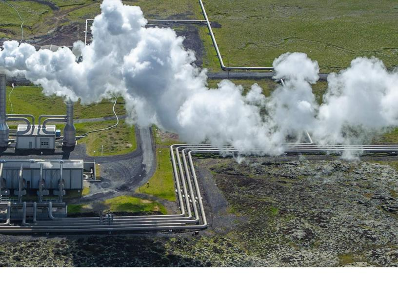
it expands into a working fluid that spins a generator to produce power. Following the process, the water is reinjected into the geothermal reservoir, while air coolers cool the working fluid before passing through the heat exchanger again. The electricity produced is integrated into the power grid for customers to use.
