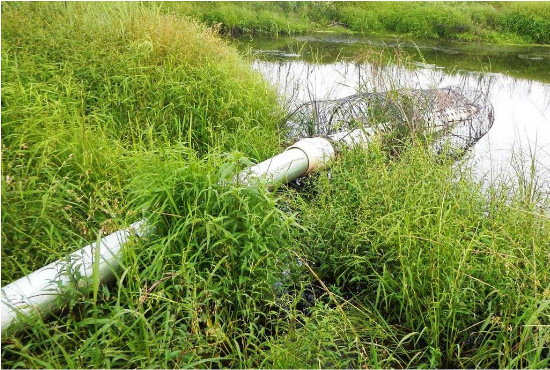
Figure 16: A “beaver baffle” ready for installation by DUC. This device reduces the ability of beavers to plug the control structure with vegetation.
