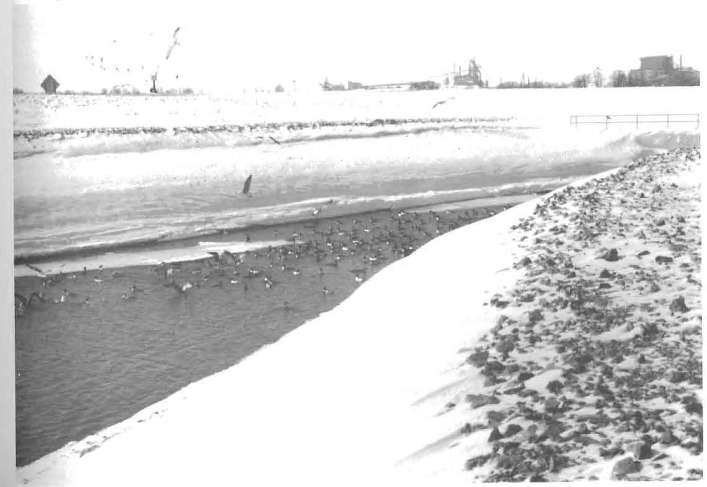
Figure 3 Waterfowl and gulls in the intake forebay of the Ontario Hydro Nanticoke Generating Station, Lake Erie, Ontario, February 1978
