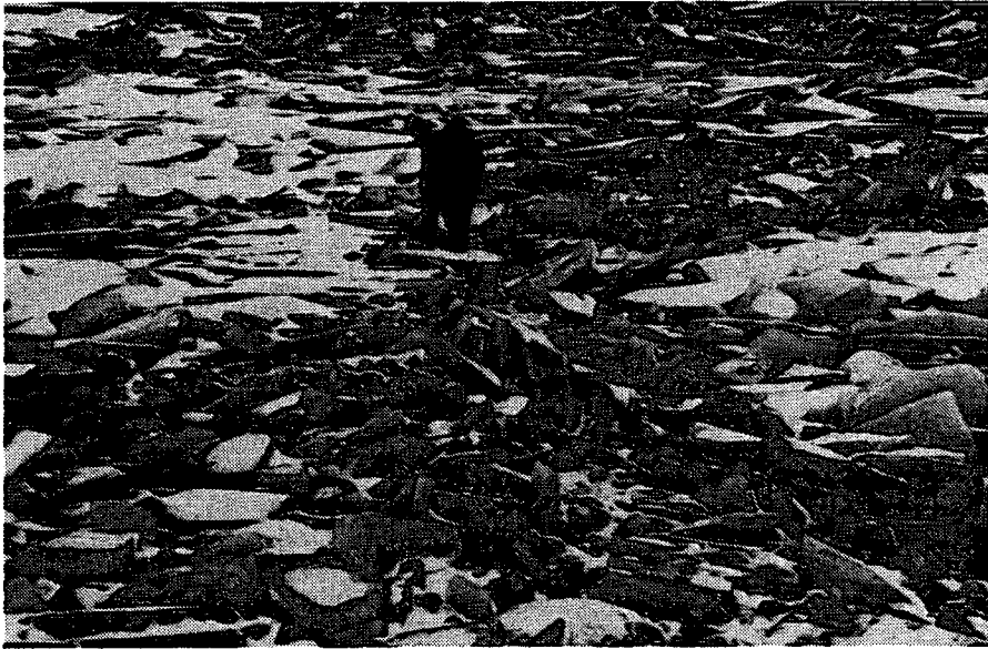
Photo 8. Preparing to drill near CP Railway Crossing. February 1986,
