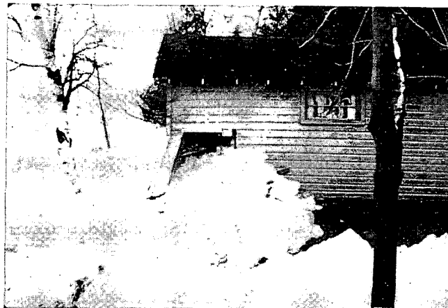
Figure 2. Cottage damaged by ice piling at Lake Simcoe.
