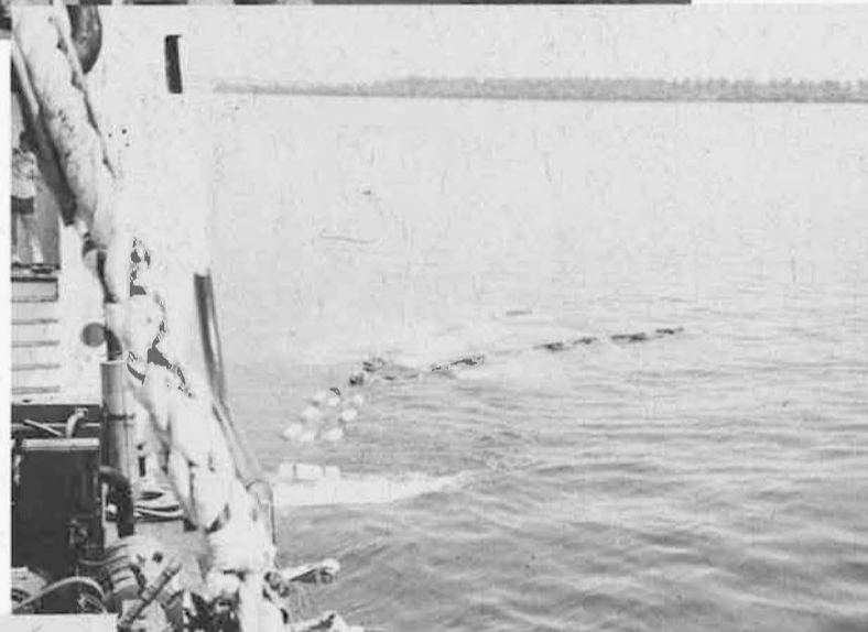
Photo 1 Manoeuvring the Barrier Into Position
