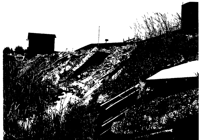
Destruction of habitat from indiscriminate filling and dumping (photo: Gary L. Williams/G.L. Williams and Associates)
