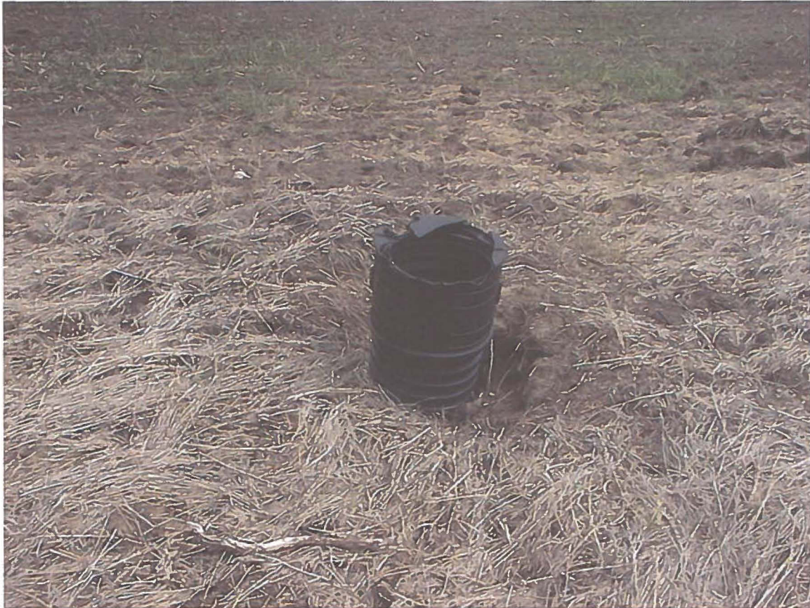
Figure 9. A 12 inch diameter drainage tile head, located in the deepest portion of what was a shallow marsh wetland. Alberta, 1999.
