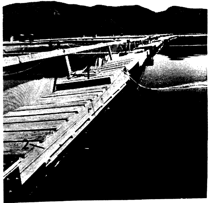
Plate 5-1: Electric fence around a salmon farm: lines around netpens (1) and walkways (2).
