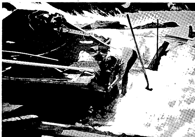
Figure 8(b). A-frame hut crushed by snow avalanche in 1967.
