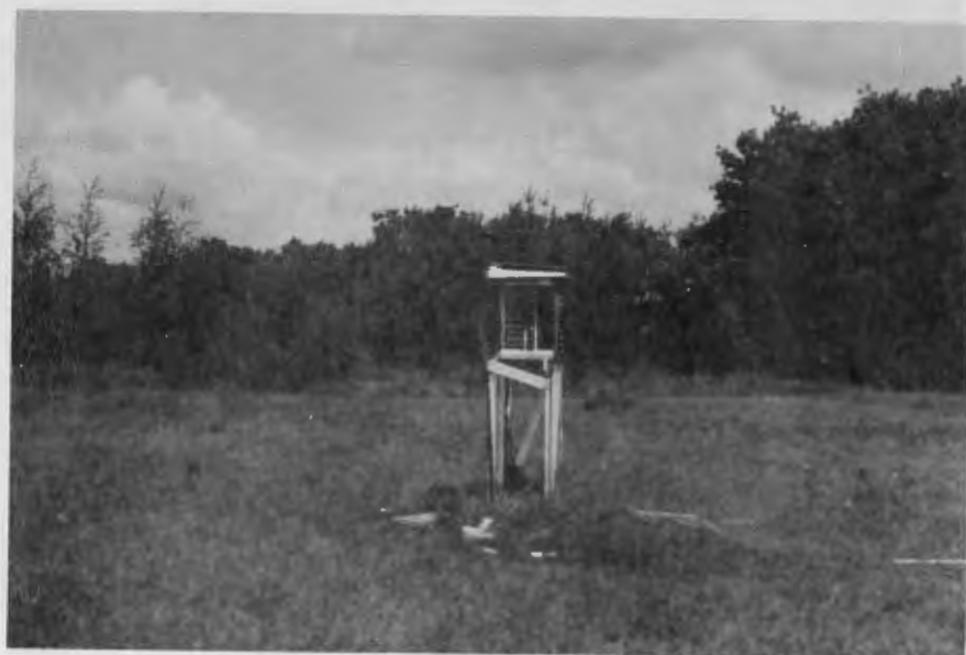
plate 3 - Looking E. General damage and scattered debris.
