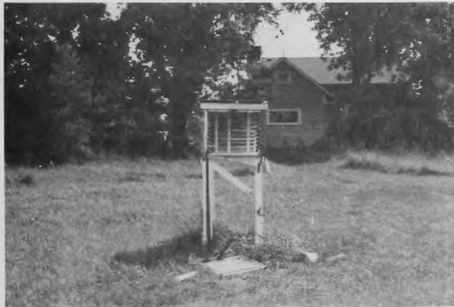
plate 2 - general damage. Dwelling and 40' maples in background. Looking S.
