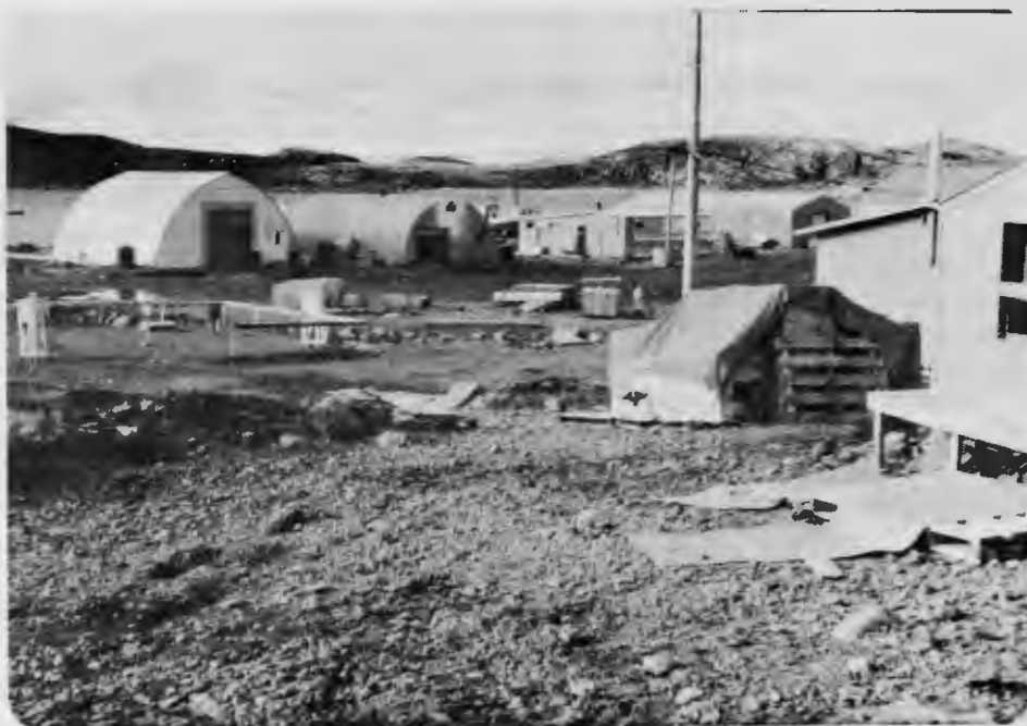
Cape Dorset Weather Station office at extreme right; meteorological instrument compound at left - 12 September 1974.
