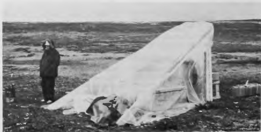
. . . the need for a messhall was not anticipated. The constant swarm of blackflies necessitated the hasty construction of one.
