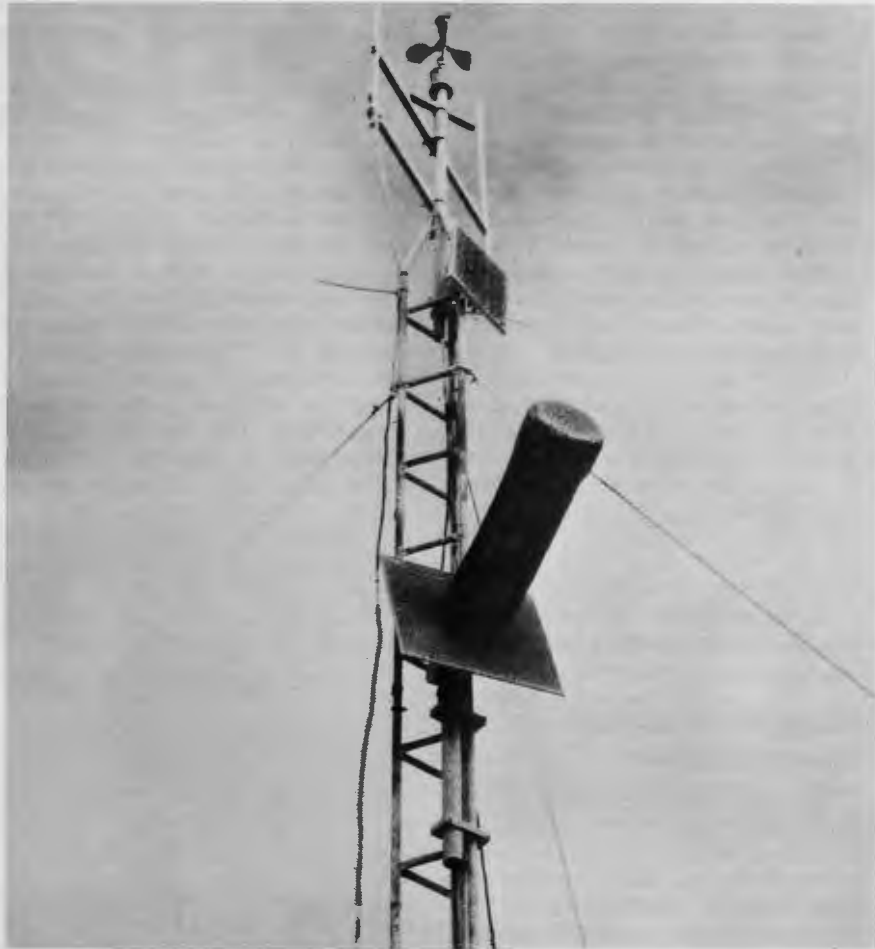
The MAPS R automatic weather station tower holds two unconventional pieces of equipment; a cylindrical antenna for broadcasting data to a geostationary satellite and, above it, a square plate holding the several circular solar energy cells which power the station.
