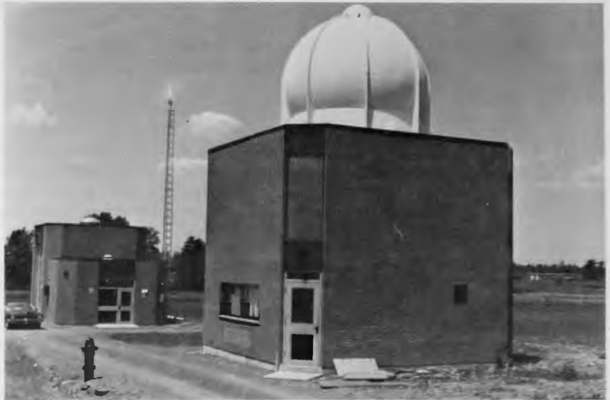
The two new Aerological Observer Training Unit buildings at Cornwall. The one with the dome protecting the receiving antenna is used for the processing of data. The building in the background contains the hydrogen generating equipment and an area to fill the balloon.
