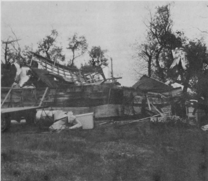
A tornado severely damaged this Yorkton, Sask. farm.
