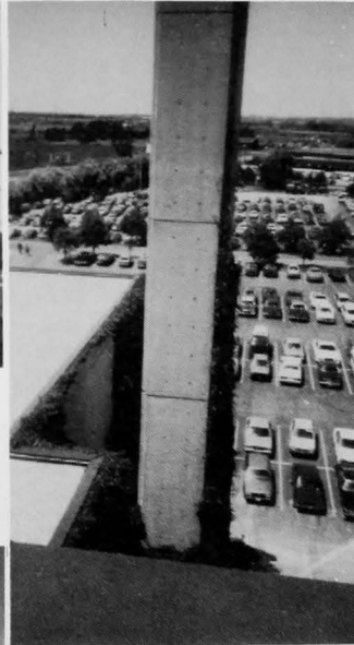
Ensclosed in the north east corner is this huge 45 metre chimney acting as the main exhaust for the boiler room. Its principal charm is the creeper plant winding its way up the side.
