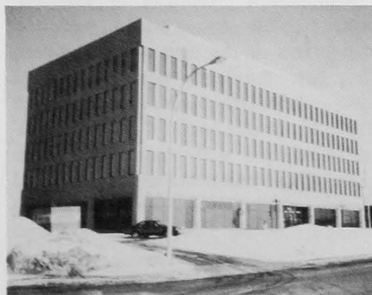
General view of the CMC building, Dorval, Que.
