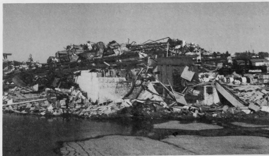
Two industrial sites west of Highway 400 in Barrie were reduced to utter rubble.
