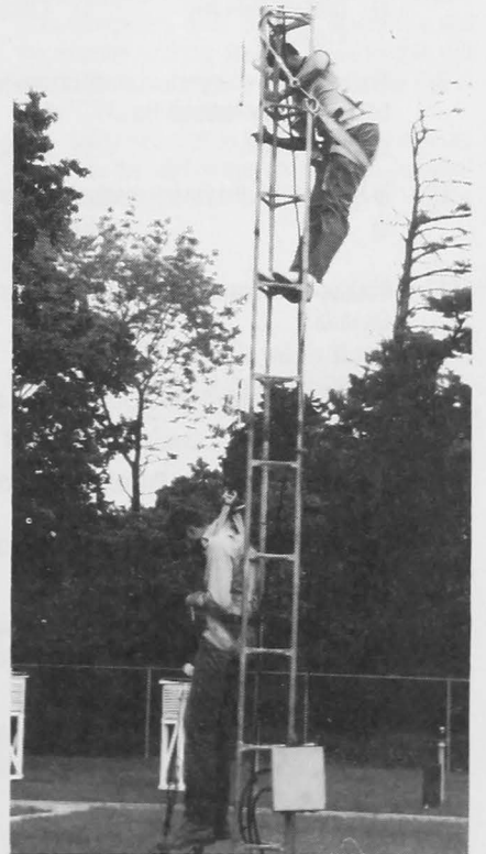
AES staff test new safety harness on standard instrument tower
