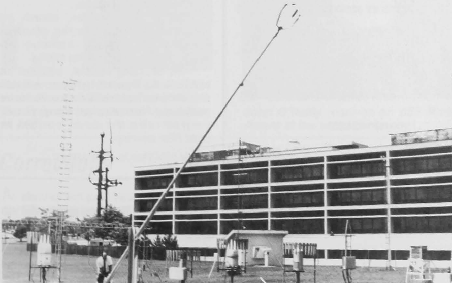
New bending tower allows instrument to be lowered to the ground
